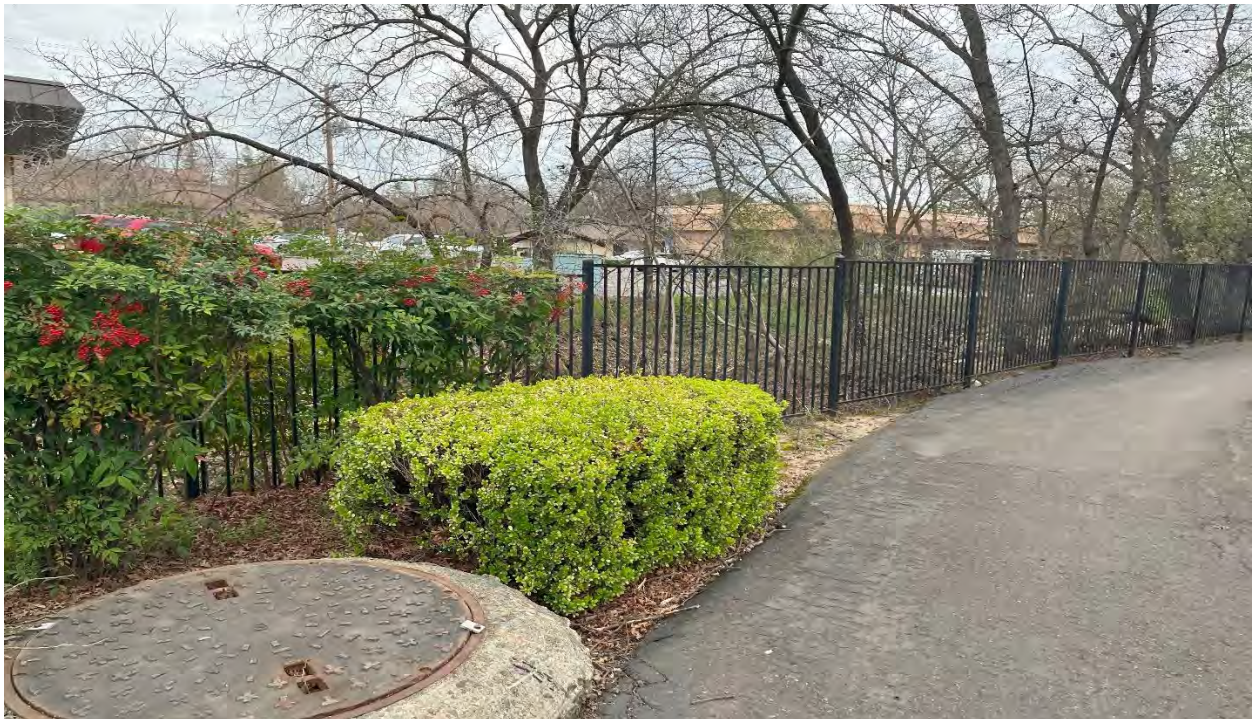
Photo 2: Northeastern corner of the subject parcel with an existing sewer line that contains a 10-foot easement. Cirby Creek is located on other side of the fence.
